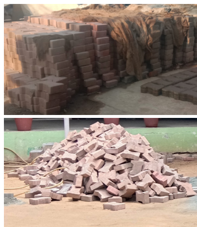
Typical stacking, curing and unloading view
